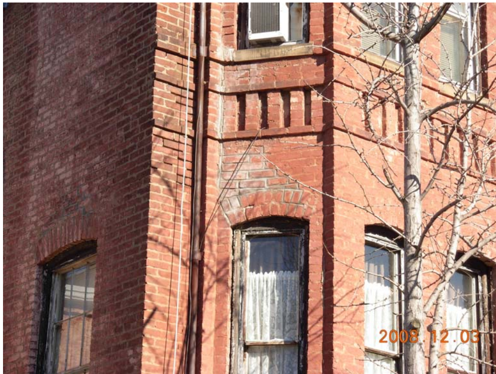
Photo 2: Step cracking, previous patchwork and deteriorated mortar at southwest bay window
