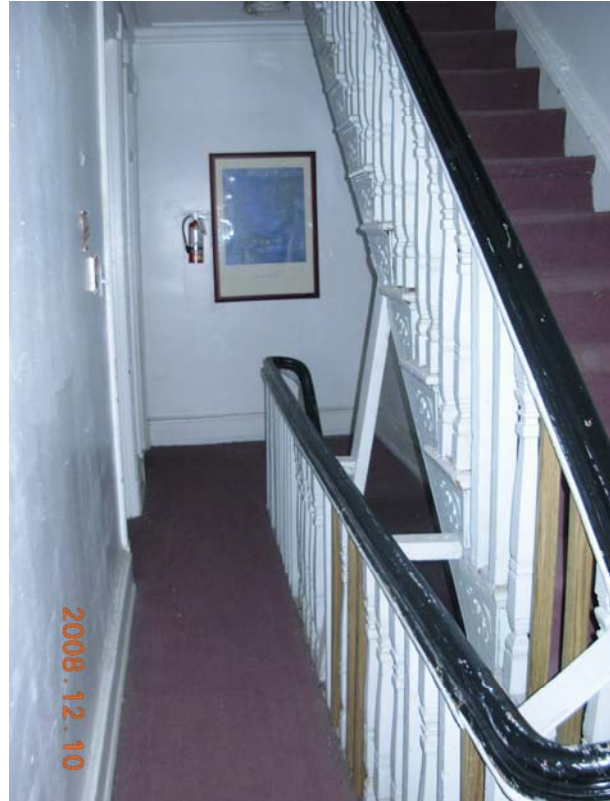
Photo 6: Handrail at third floor with previous repairs
