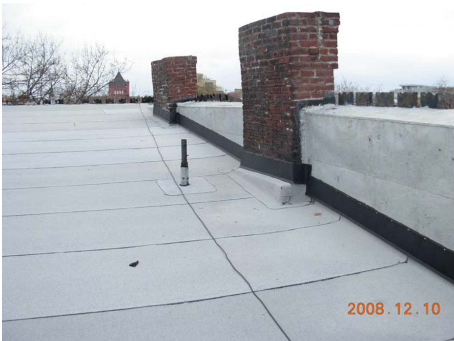
Photo 7: Roof, chimneys, parapet with partially deteriorated metal scallops
